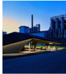
Zeche Zollverein Essen (Germany) Project: Lighting Design: Engineer Büro Paulus Essen, Herr Gräf
