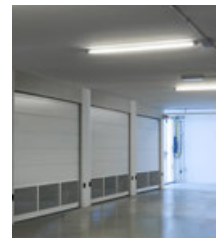
Residence Civico 3.9 Castelfranco Veneto (Italy)
