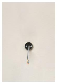
Thread the wires through and fasten the multiple rose support.
