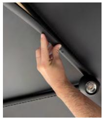
Applying the cover to conceal the exposed parts of the electrified track module.
