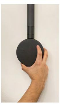
Complete the operation by tightening the rose element in a clockwise direction.
